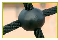
8- The 16mm diameter ropes are made of galvanised steel cable covered with polyester. The cables are linked together and held in place by injected polyamide spheres.
