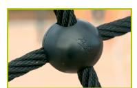
**3- The 16mm diameter ropes** are made of galvanised steel cable covered with polyester. The cables are linked together and held in place by injected polyamide spheres.
