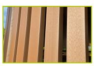
3- The slatted fences are produced using post-consumer waste, mainly recycled food and drinks containers (polyethylene, aluminium). This environmental impact reducing material is an inert and robust compound which is hard-wearing, resistant to UV light and fluctuations in temperature, and able to retain its shape over time. It is also rot-proof, making it a reliable option for outdoor applications.
