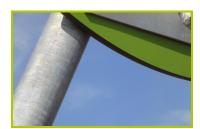
**10-The support legs** are made from 60mm galvanised steel.
