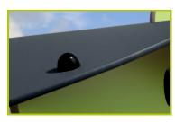
8- The roof is made of 10mm thick polyethylene plates.
