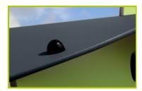
**3- The roof** is made of 10mm thick polyethylene plates.
