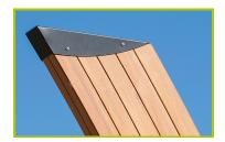
**2- The shaped beams** (95mm thick, 200mm wide and 3.2m high) are made of oven-cured laminated wood with a surface coating; It gives the structure considerable strength.
