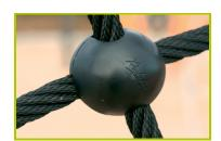
**8- The cables** are linked together and held in place by injected polyamide spheres.
