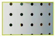
**7- The balcony** is made of 3mm perforated aluminium sheet, coated with polyester epoxy lacquer.
