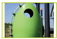
**6- The pod** is made of 4mm thick polyester. It is a durable material and this ensures its resistance to weathering and UV radiation.
