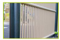
2- The mesh fencing is made of painted aluminum. The goal area mesh fencing is made of painted galvanised steel.
